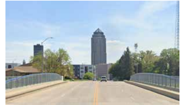
Above: The existing 9th Street Overpass can be redesigned as a welcoming multi-modal entry to Downtown as shown by the rendering on the subsequent page.
